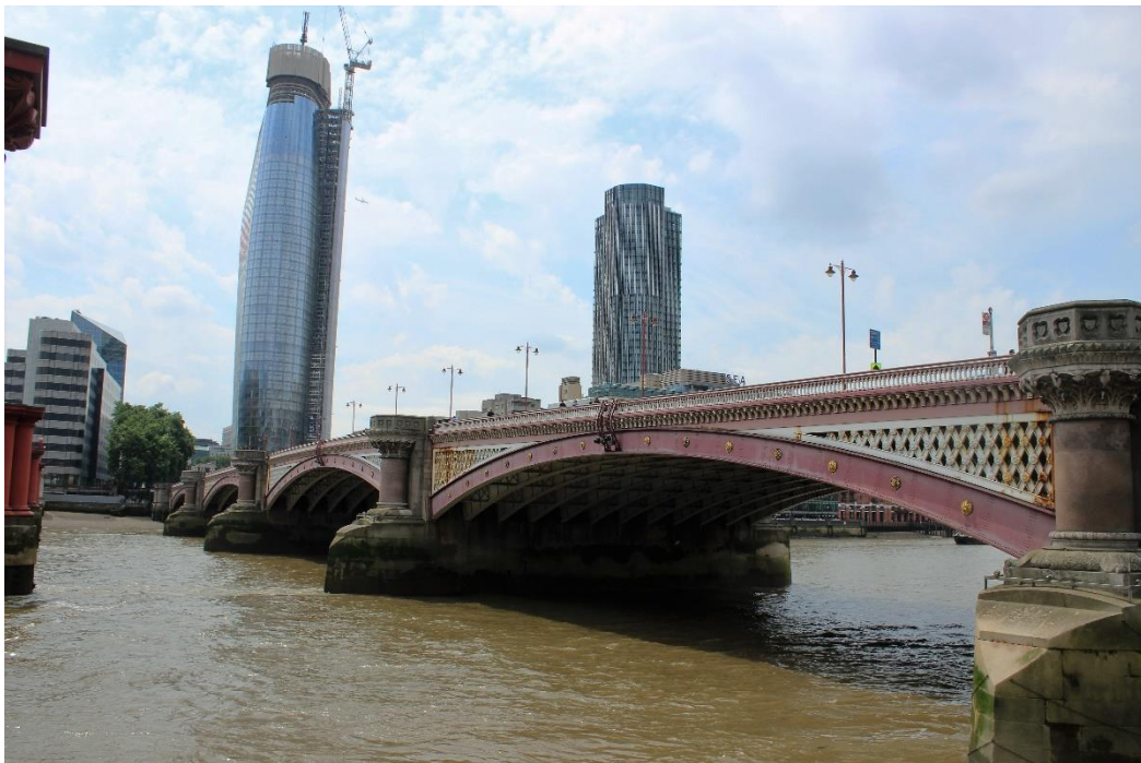
Blackfriars Road Bridge showing underside ledges suitable for roosting feral pigeon and starling ©Tony Wileman
